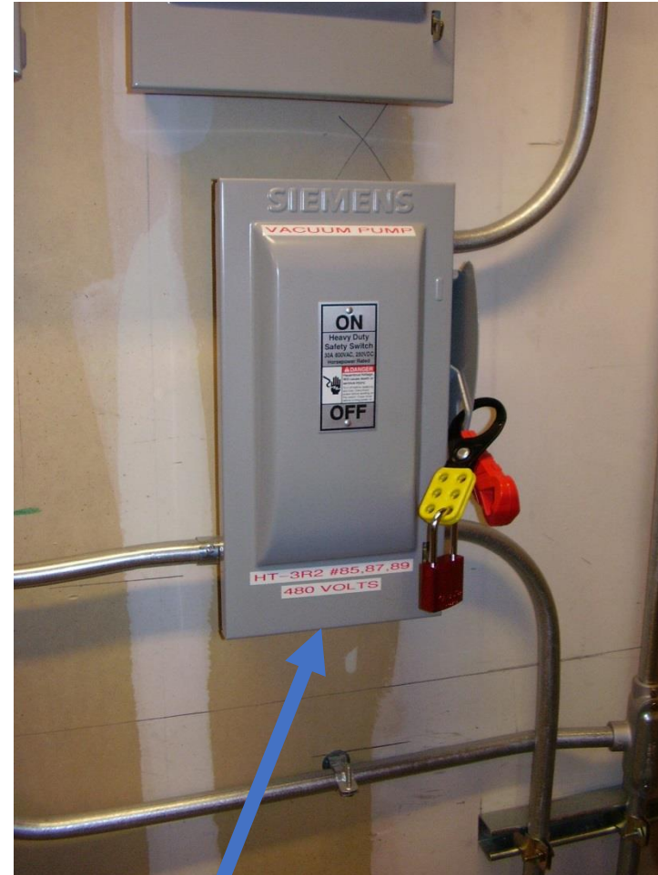
Locked Out with Hasp & Lock
