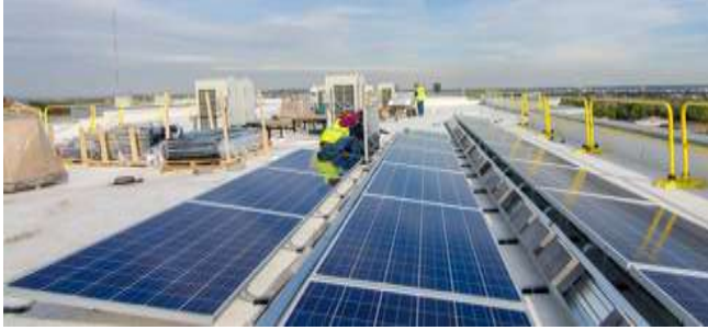
Figure 3. Celentano hall fixed modules with 12° inclination
